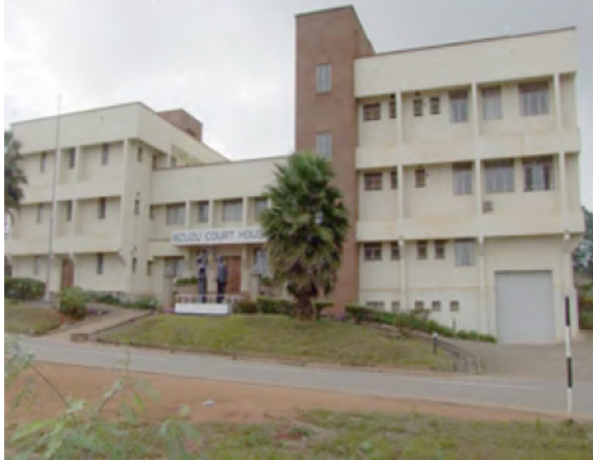
Fig 11.4: the High Court Building
